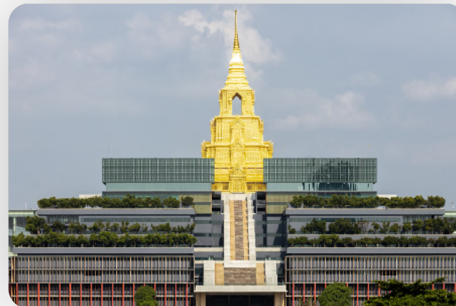
Sappaya-Sapasathan, the National Assembly of Thailand
